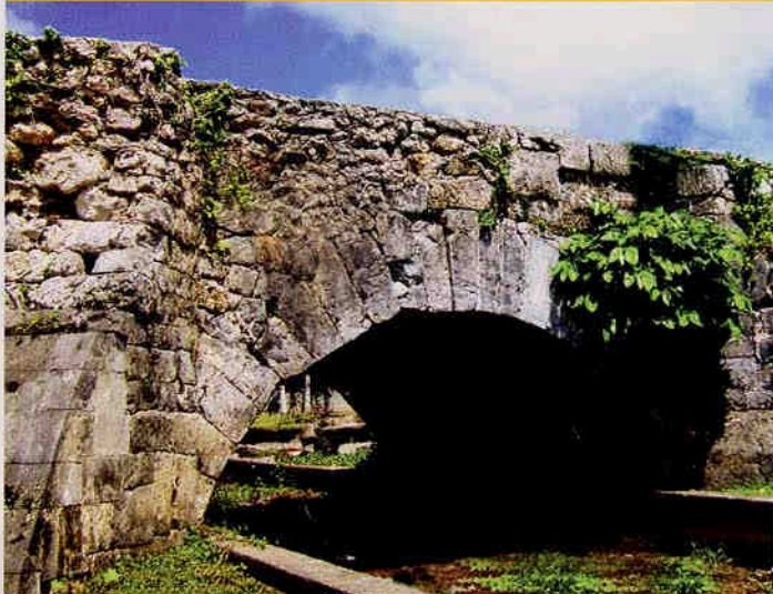
Tolai Acho (San Antonio Bridge)
